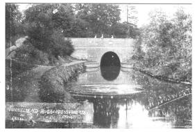
The tunnel at Husbands Bosworth is 1166 yards long and was completed in 1813. Over 2,000,000 bricks, made in a brickworks set up specially for the purpose, adjacent to Honeypot Farm Bridge, were used in its construction.
