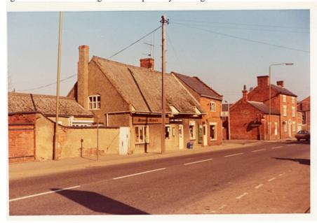
profile that can be seen elsewhere in Bosworth on the corrugated iron-roofed cottage presently being renovated at 32-34 Bell Lane and at 48 High Street, which is asbestos clad, similar to Hunters Cottage. Difficulties arranging guttering meant that thatch roofs typically have a large overhang and the guttering is usually an open gully in the pavement!
